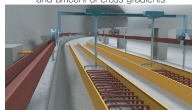
Arranging steel bars and installing molds
